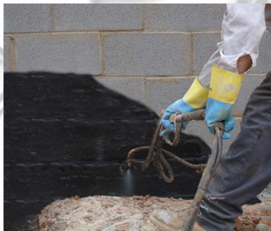
BoneDry™ RP waterproofing membrane shown with available 12" DrainMax™ foundation strip drain to make the BD1000 Waterproofing System
